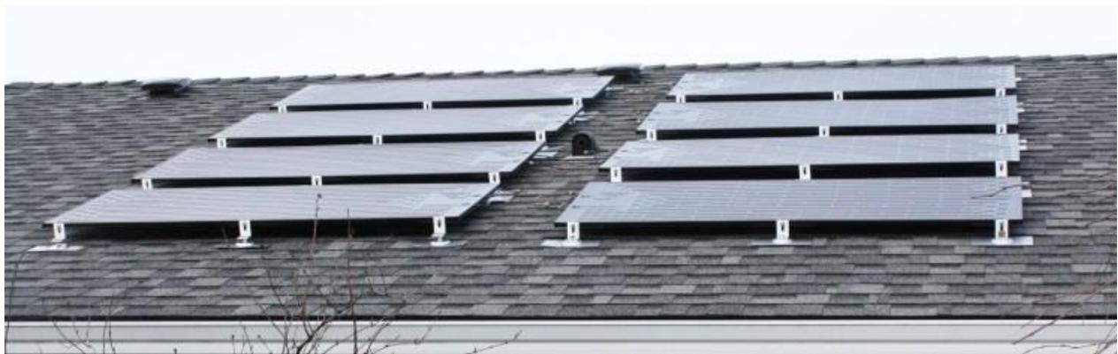
Above is a 2 x 4 Array of 8 Panels for a 14 kW SunPump on a typical asphalt shingle retrofit roof. Notice the scoop shaped pipe flashing in the center for the Line Set, as a good location for fitting the manifolds. Best is flashing location is one row down to allow for the Manifold and shortest equal length tubes.
