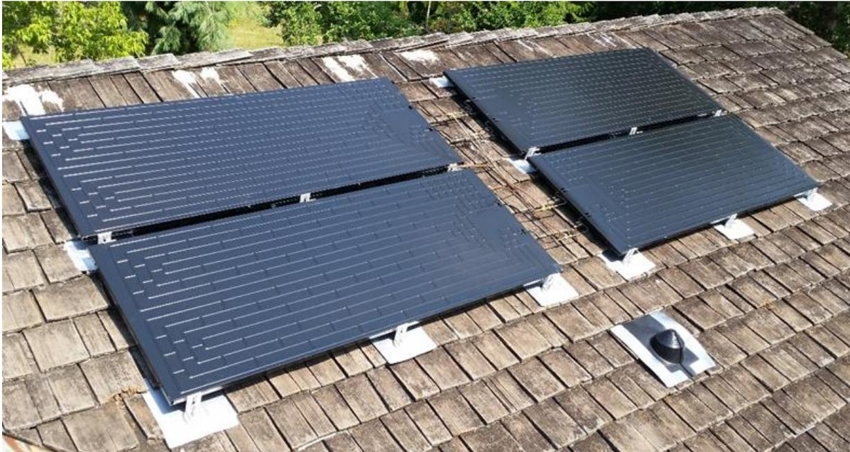
Shingle or Asphalt Shingle Roof – L-Foot Kits
