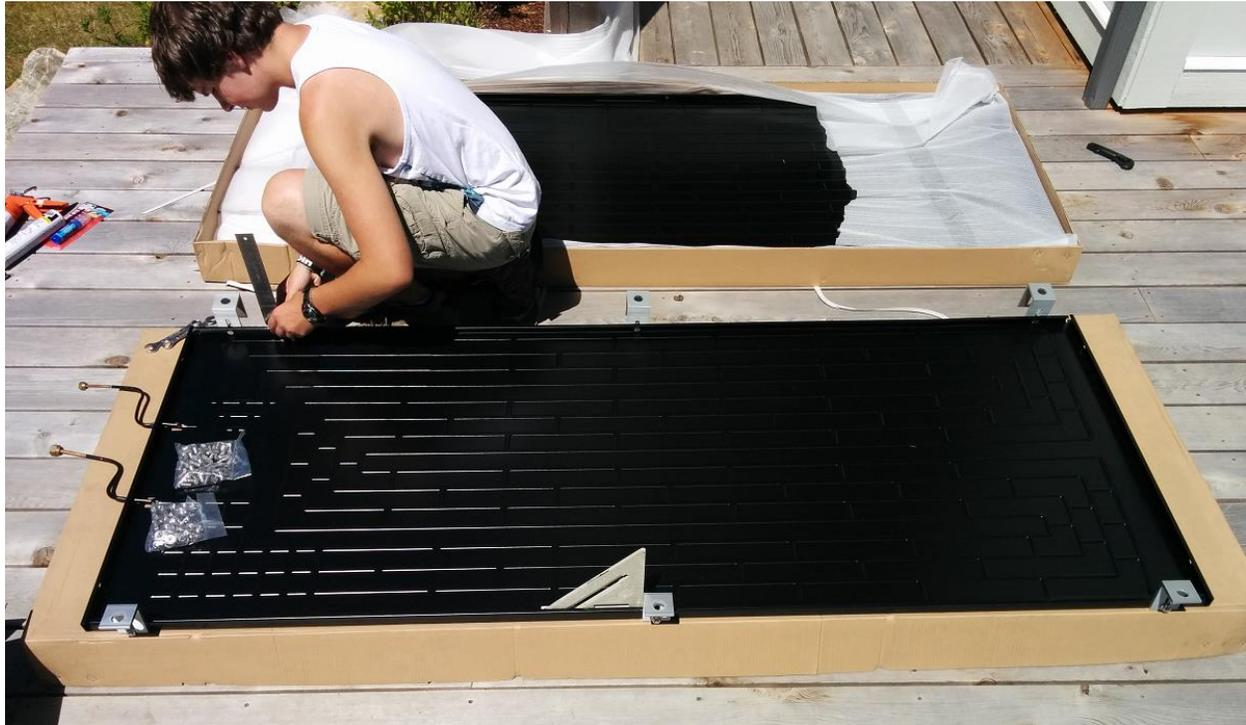
**Step 2: Attach the Defrost Sensor to one Panel.** The Panel Sensor is a NTC 10k Ohm Resistance Thermistor on AWG22 two wire.
