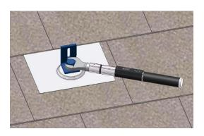
Install AL rail to "L" foot to the specific orientation. Then, tighten 3/8 flange nut to 15 ft-lbs and 1 1/16 AL hex cap to 20 ft-lbs torque.
